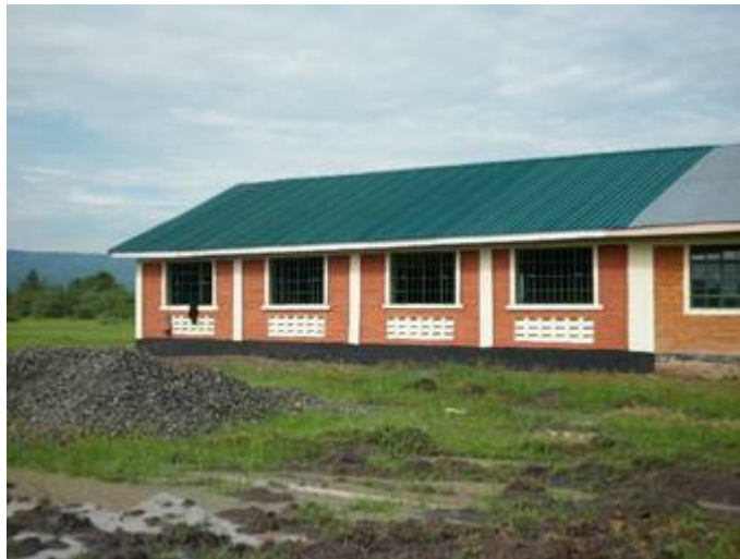
Hannah's Hope Phase III Construction
