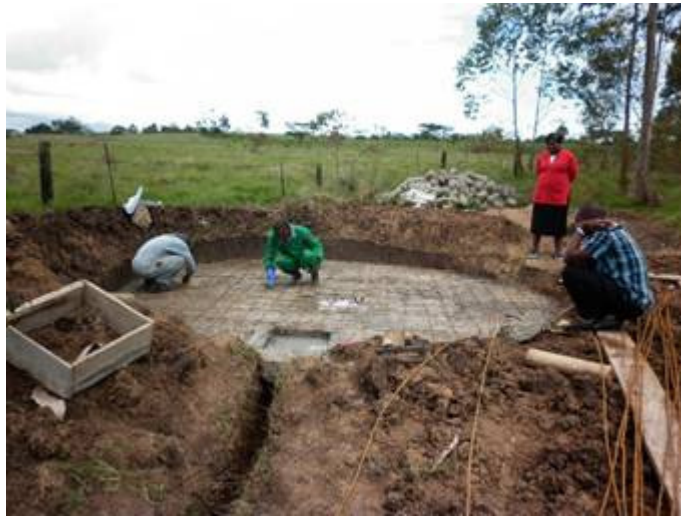
Beginning of Construction of Water Storage Tank at Kongasis
