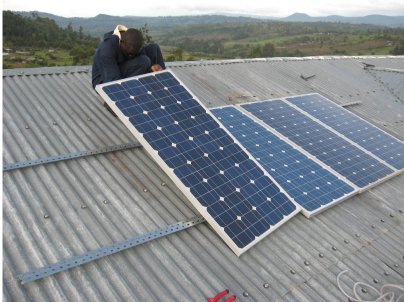
Solar Panels being installed at Kongasis
