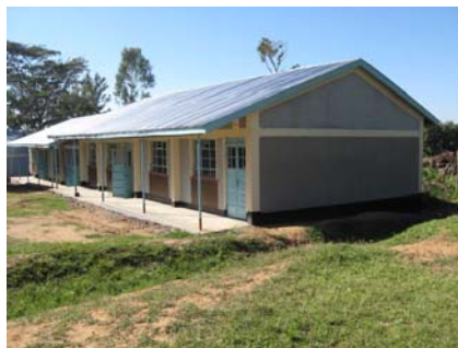
Lufumbo Classrooms Near Completion
