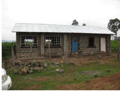
Kongasis Kitchen Just Prior to Completion
