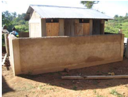
Iranda Latrines Under Construction
