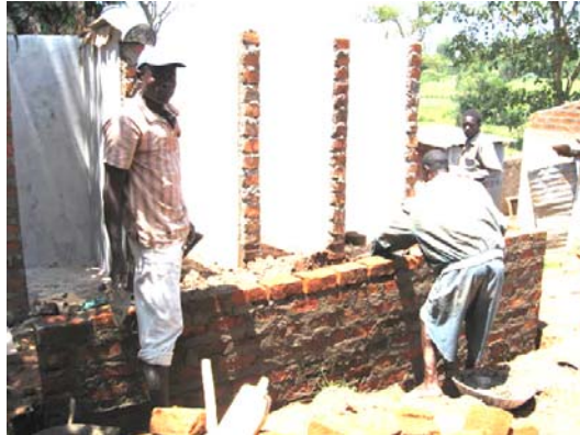
Iranda Latrines Under Construction
