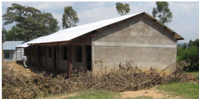
Lufumbo 4-Classroom block under construction
