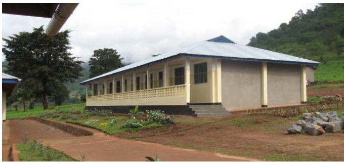
Joining Hearts and Hands just finished the construction of these three Usambara classrooms!
