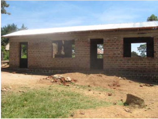
Iranda Kitchen Under Construction
