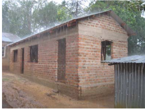
Lufumbo Kitchen Under Construction
